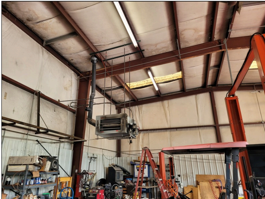
6 - Used oil heater in maintenance area
