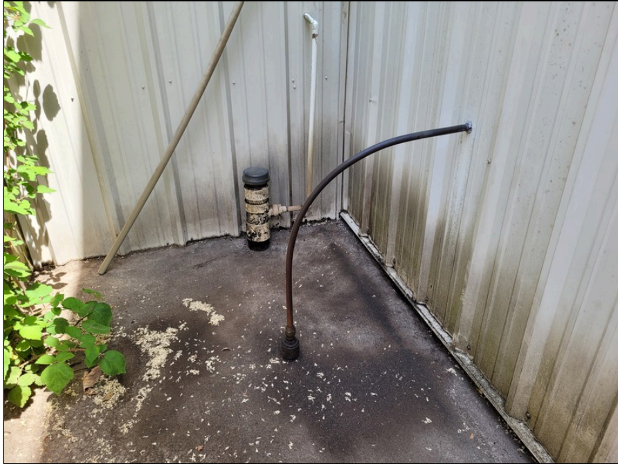
21 - Used oil UST vent pipe
