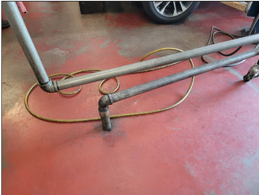
4 - Used oil pipe in maintenance area
