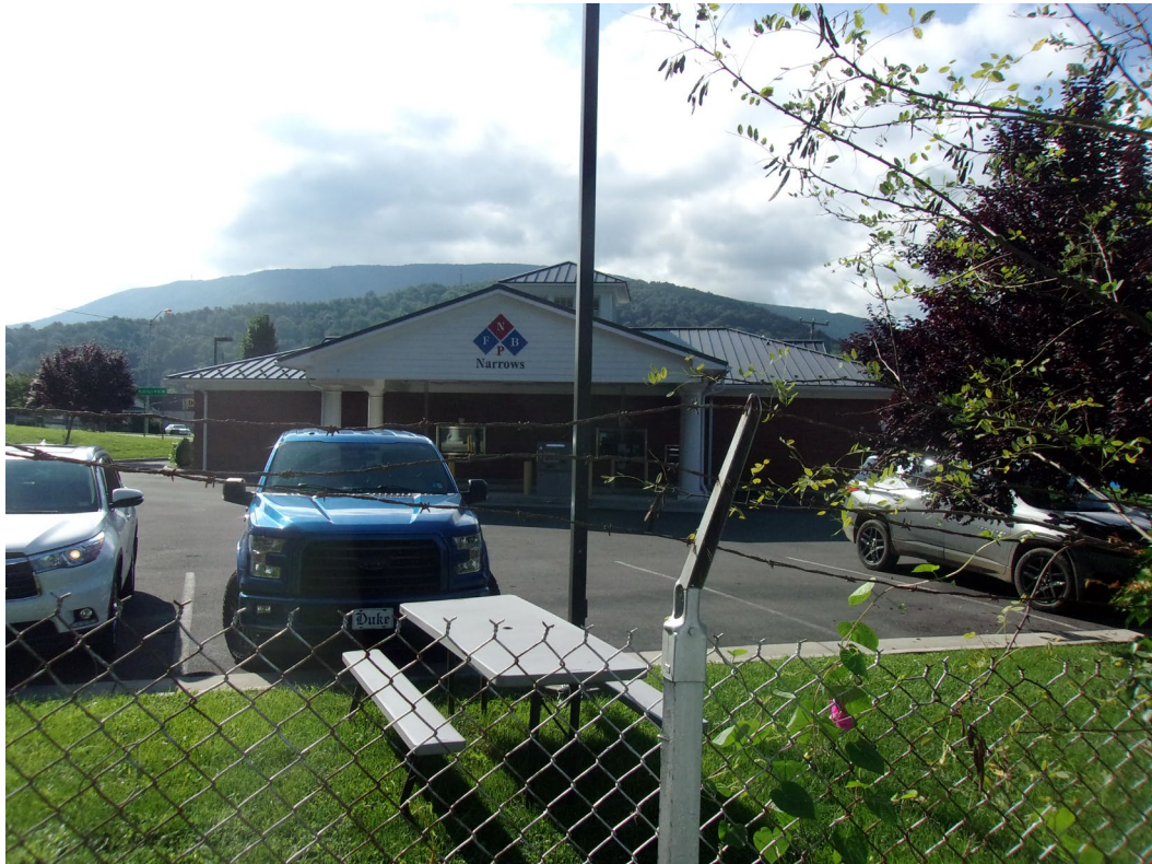
Photo #5: View of the eastern adjacent property. Photograph taken facing south.
