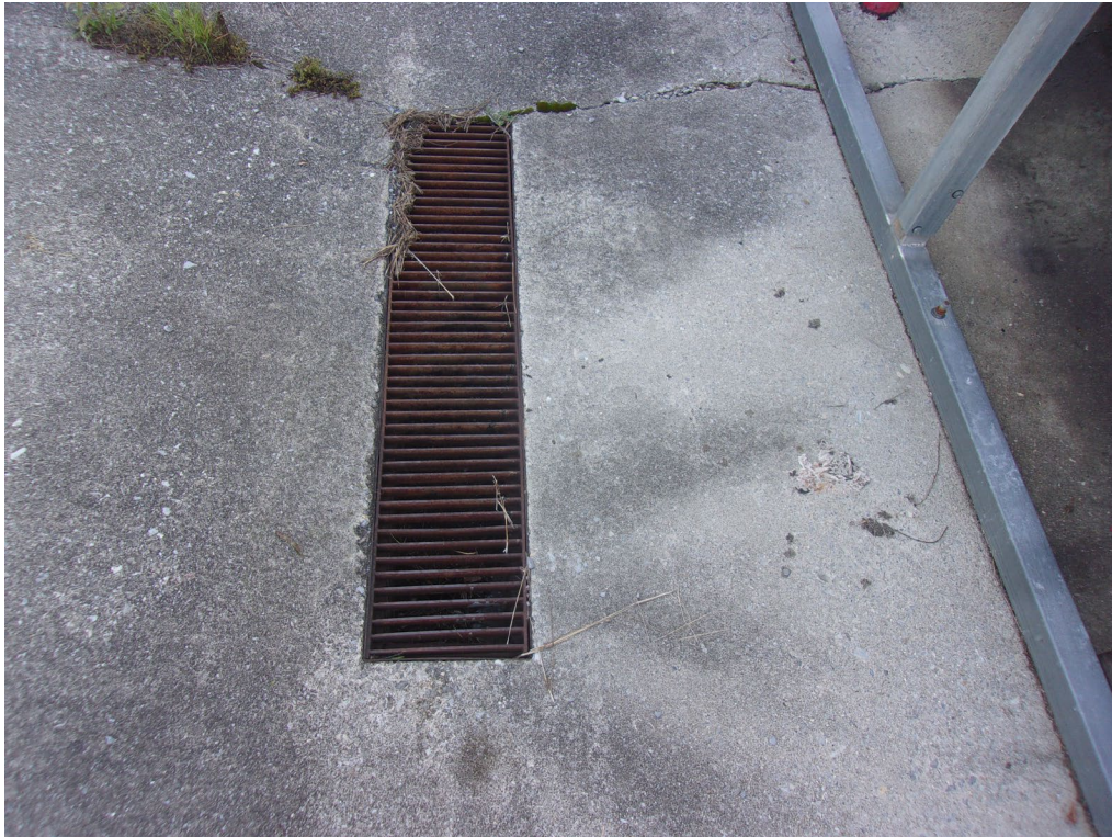
Photo #9: View of the trench drain.
