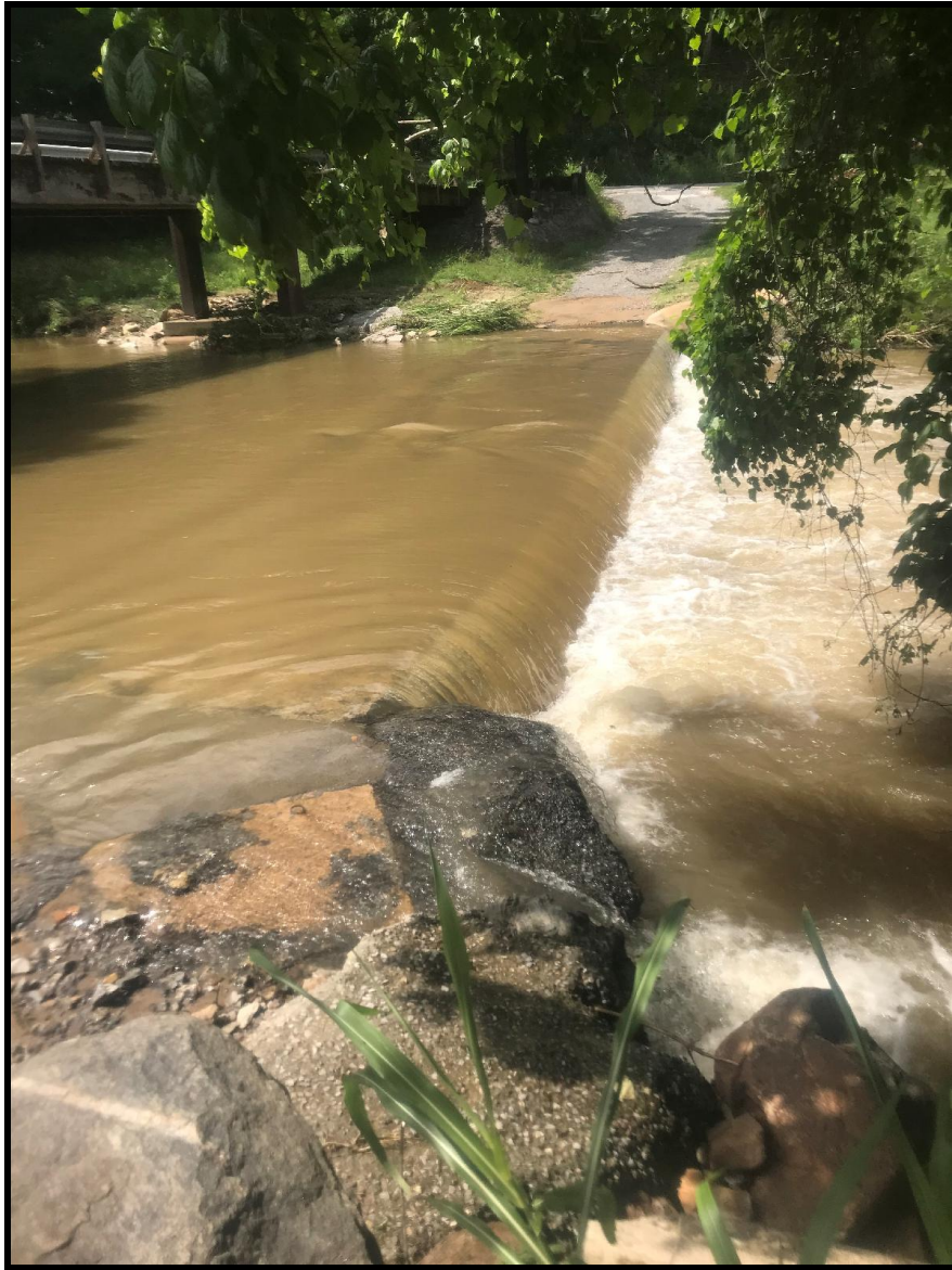
Photo 3: Low water bridge crossing of Back Creek at entrance to the Ferguson Tract.
