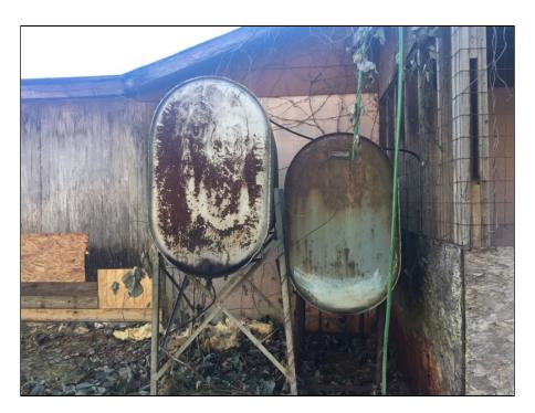
7 - ASTs for diesel fuel for the generator.
