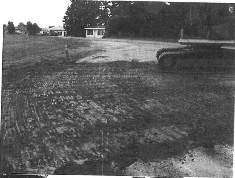
View showing diesel/kerosene tank pit backfill being compacted by excavator roll-over.
