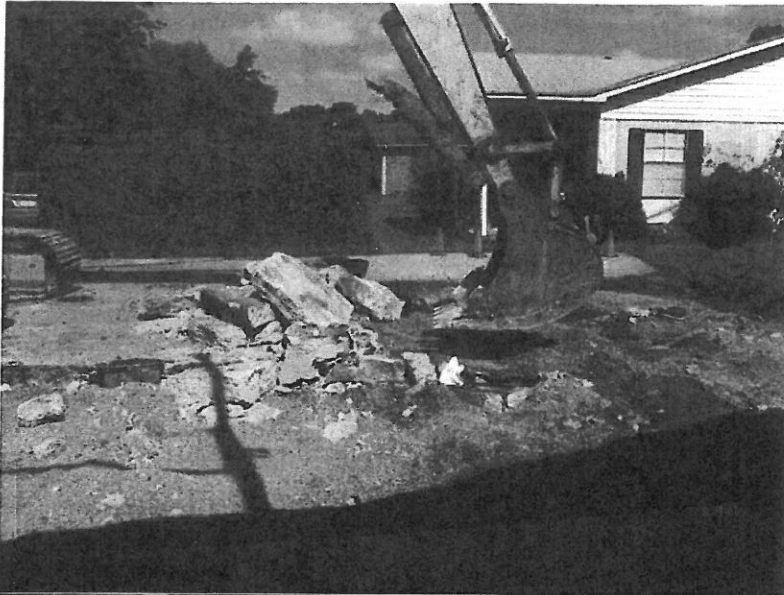
Concrete pad removal over gasoline tanks.
