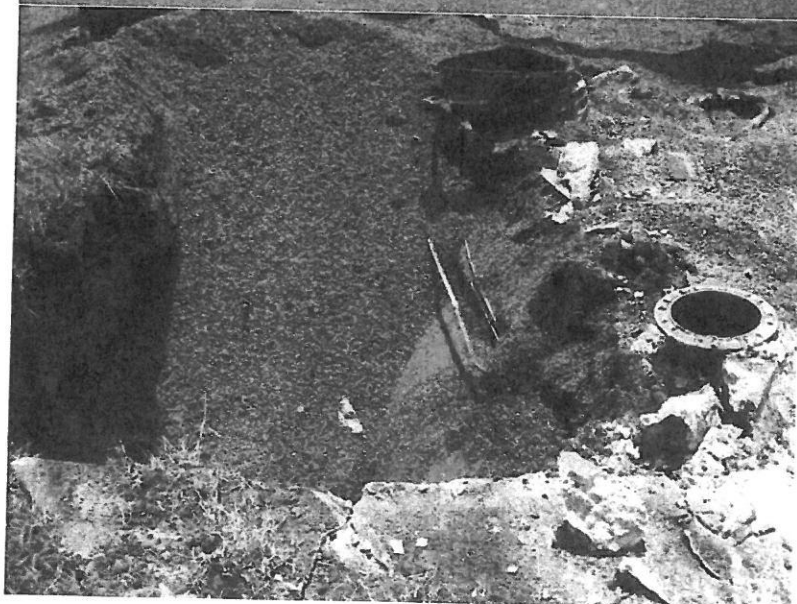
View of first exposure of diesel/kerosene tank with pea gravel overburden.
