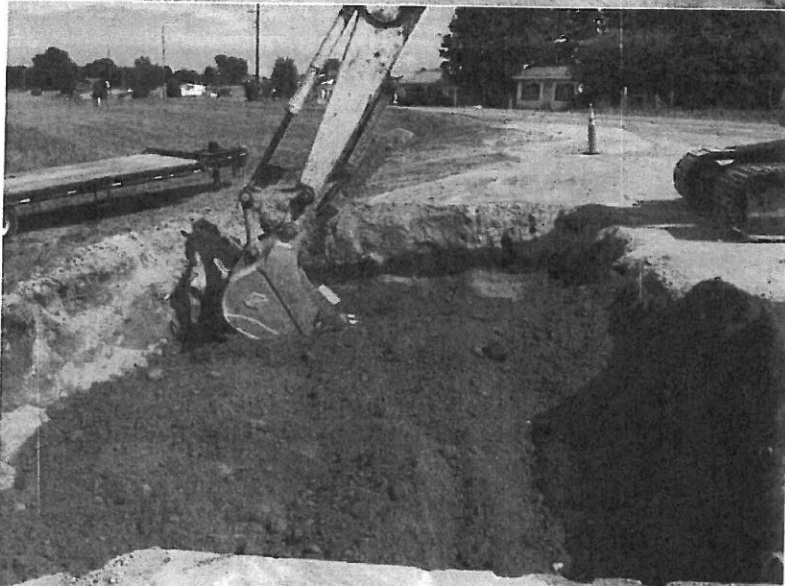
View showing diesel/kerosene tank pit being backfilled with clean, red clay fill.
