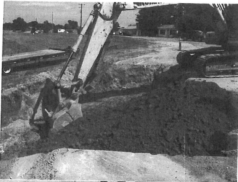
View showing diesel/kerosene tank pit being backfilled with clean, red clay fill.
