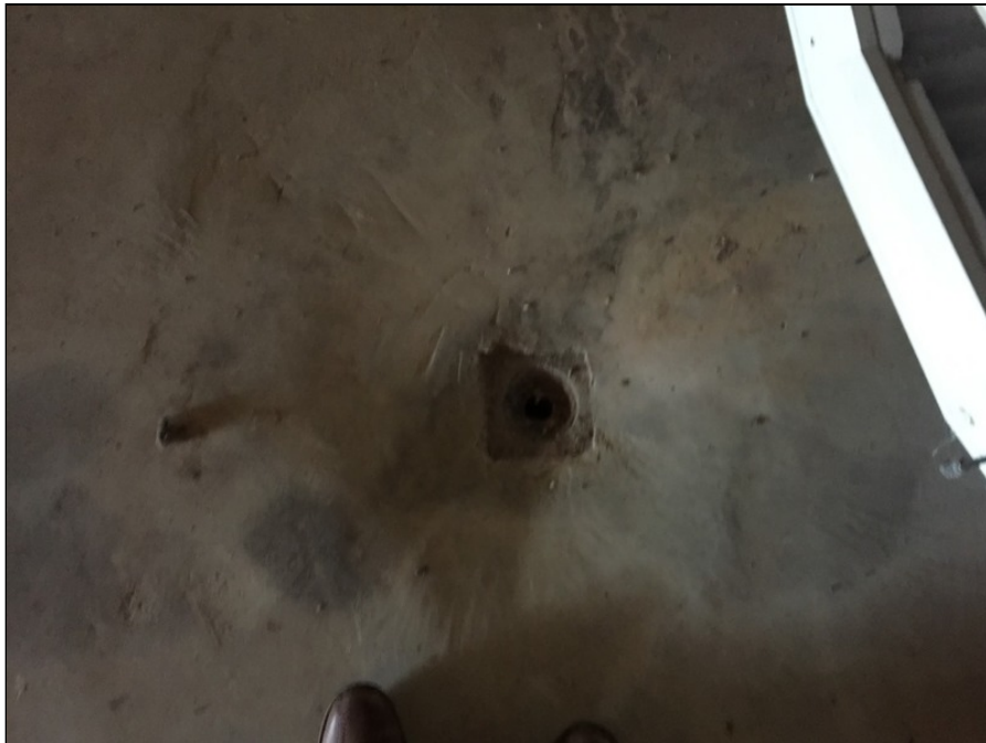
12 - Floor drain within the basement of the convenience store.
