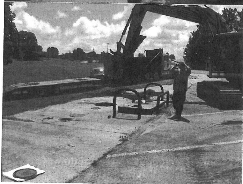
View of beginning of concrete pad removal over diesel/kerosene tank.
