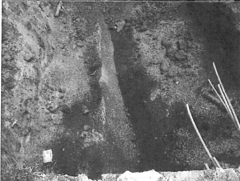
View showing diesel/kerosene tank pit bottom with pea gravel and sandy clay saprolite native soils.
