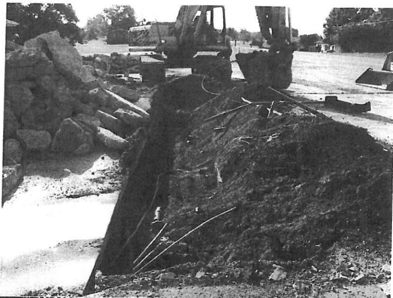
View showing gasoline dispenser pump island after excavation.
