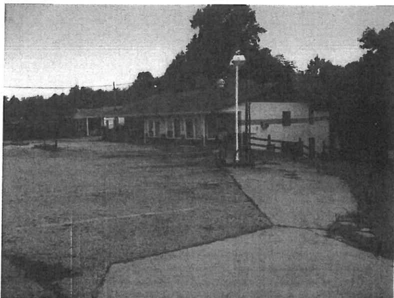
View across site prior to UST removal work looking at diesel/kerosene tank location on east side of property.
