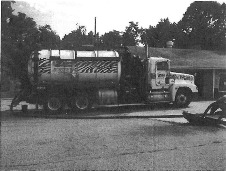
View of vacuum truck at start of product line evacuation for gasoline lines.
