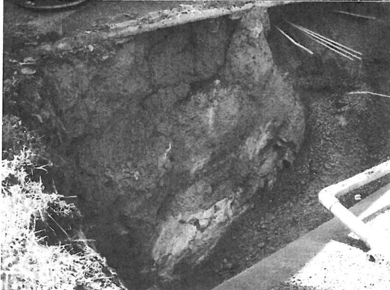
Good view of native sandy clay saprolite in excavation sidewall.
