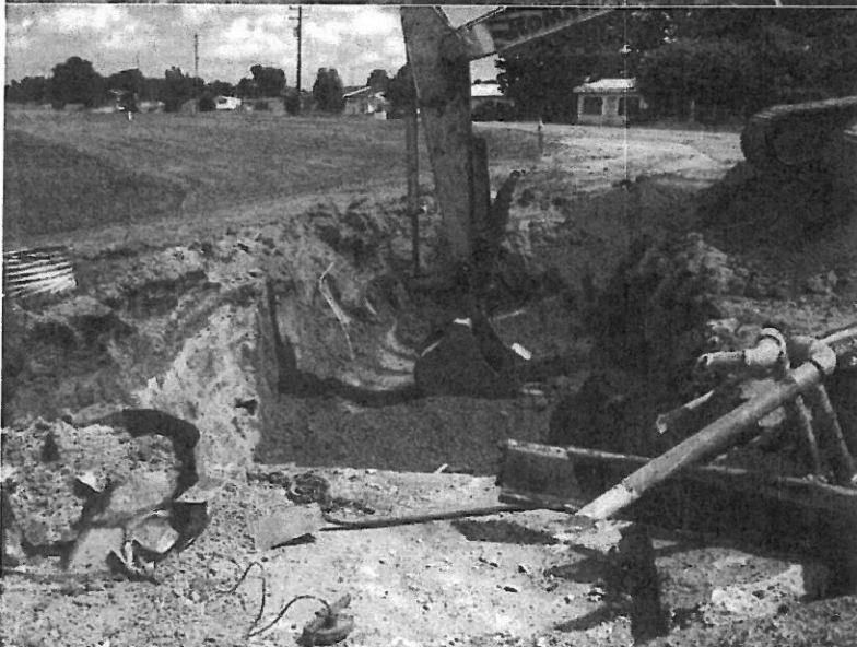
View showing diesel/kerosene tank pit being backfilled with overburden.
