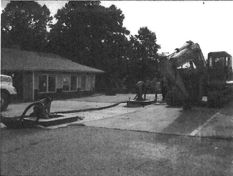
View of gasoline product line evacuation.
