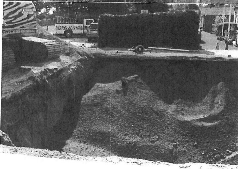
View showing backfilling of gasoline tank pit with pea gravel overburden.
