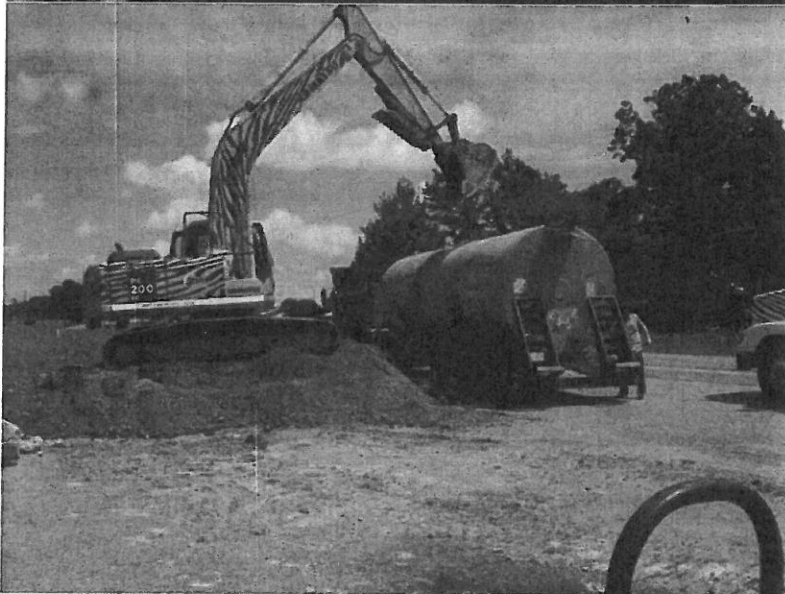
View showing diesel/kerosene tank being loaded for disposal transport from site.
