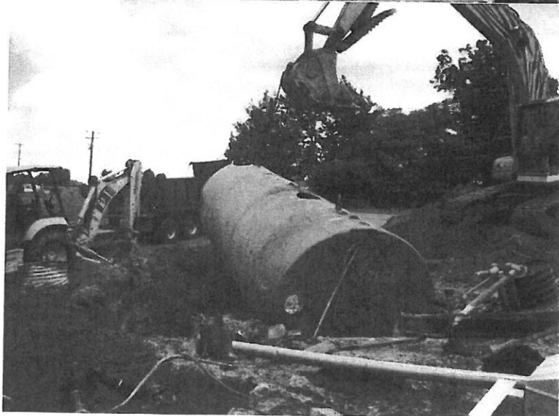
View showing diesel/kerosene tank being hoisted from pit.
