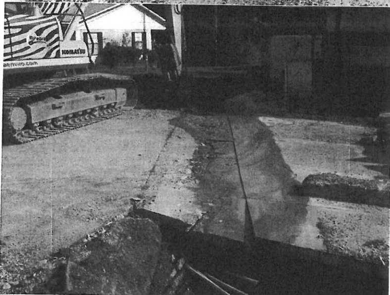
View showing saw cut of concrete over gasoline product line trench.
