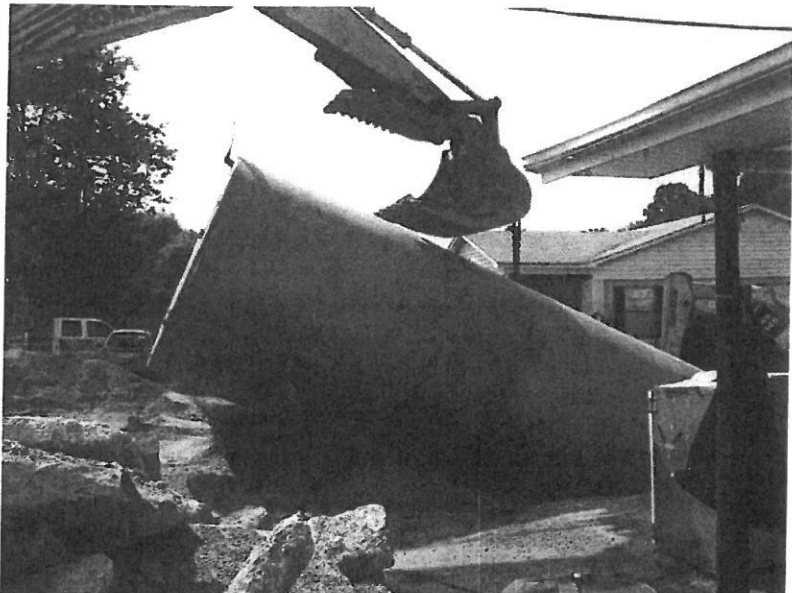
View showing second gasoline tank being hoisted from tank pit.
