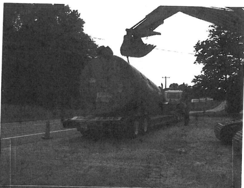
View showing first gasoline tank being loaded for transport.
