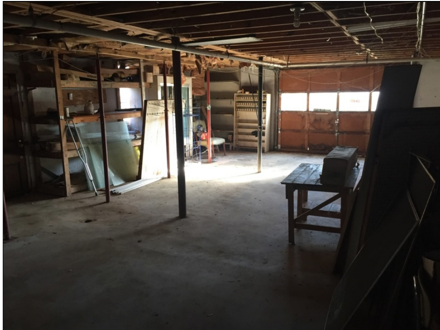
15 - Storage area in the basement of the convenience store.
