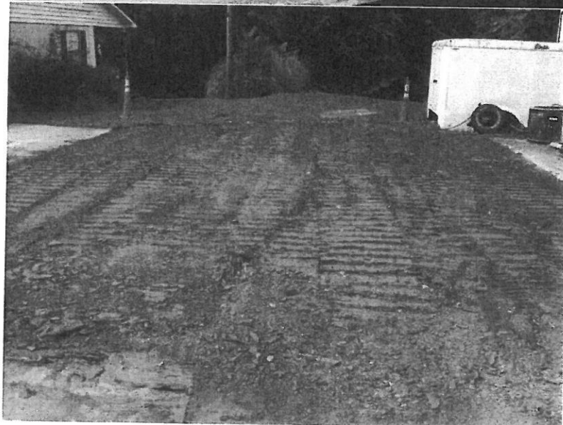
View showing gasoline tank pit after backfill and compaction with clean, red clay soil.
