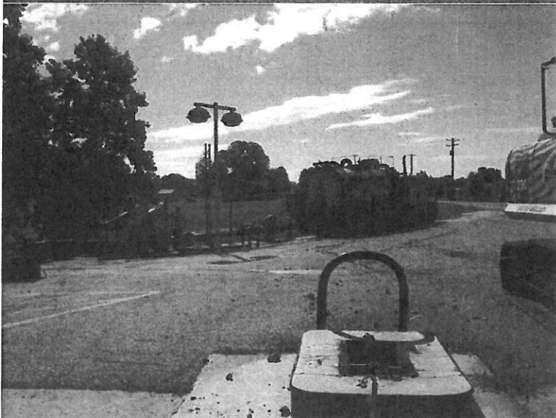
View diesel/kerosene product line evacuation.
