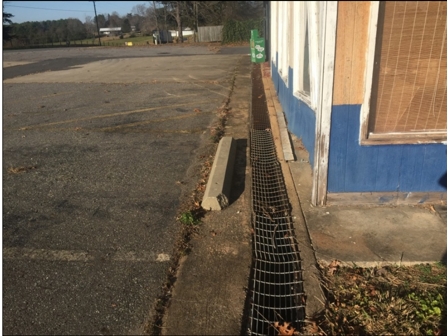
5 - Drain in front of the convenience store.
