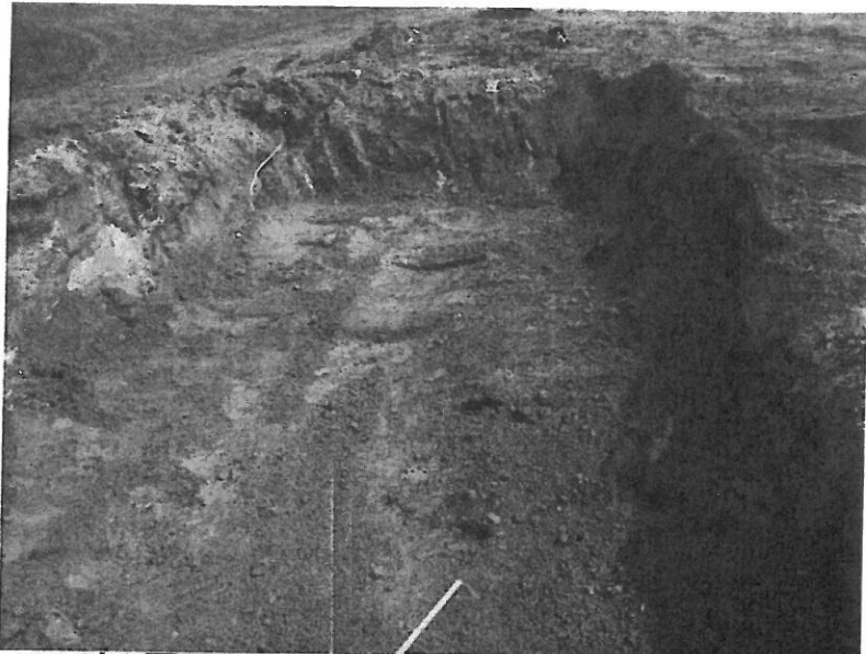
View showing diesel/kerosene tank pit bottom following backfill with overburden soil and pea gravel.
