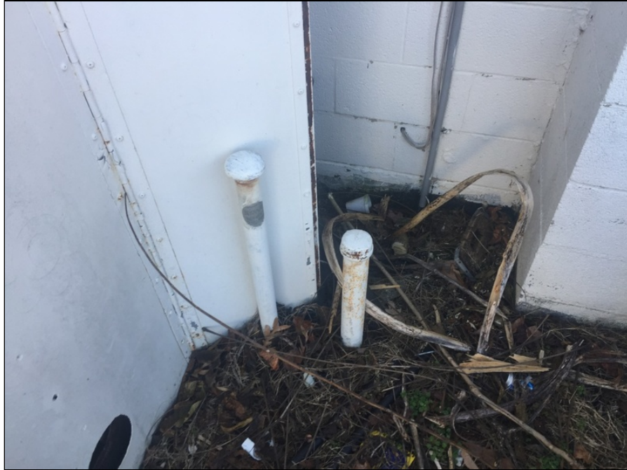
3 - UST fill port and vent pipe for the convenience store, located near the western portion of the property.
