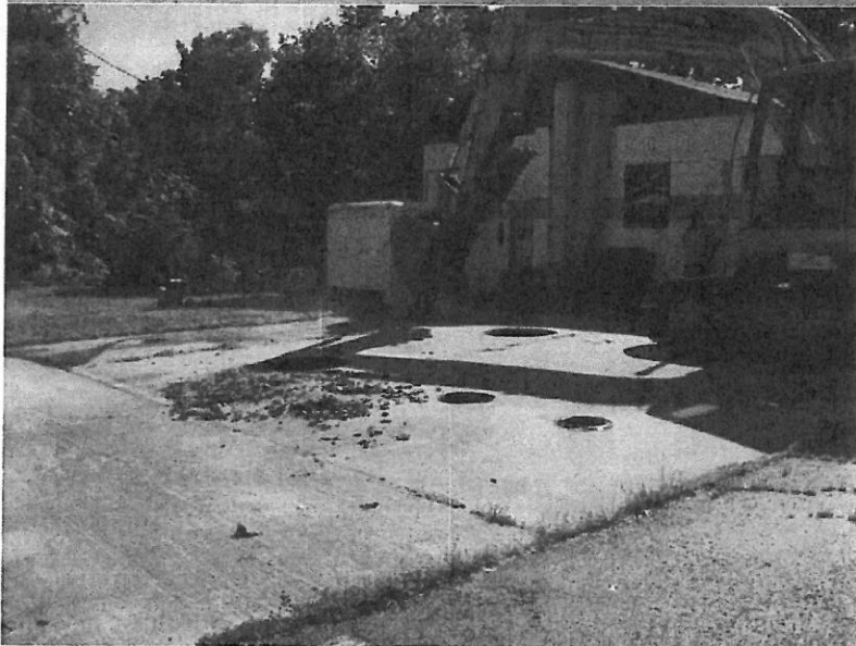
Beginning of concrete pad removal over gasoline tanks.
