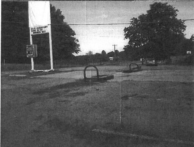
View of former gasoline dispenser pump locations.
