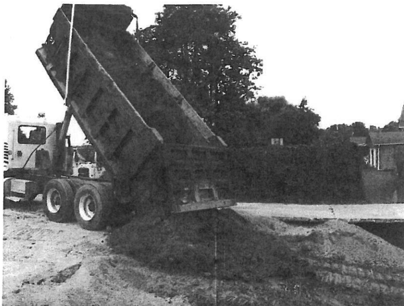
View showing gasoline tank pit being backfilled with clean, red clay soil.
