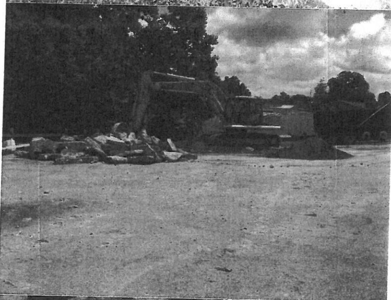
View showing beginning of diesel/kerosene tank excavation following removal of concrete pad.
