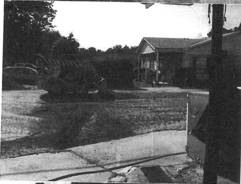
View showing top layer of ABC stone being spread over gasoline tank pit.
