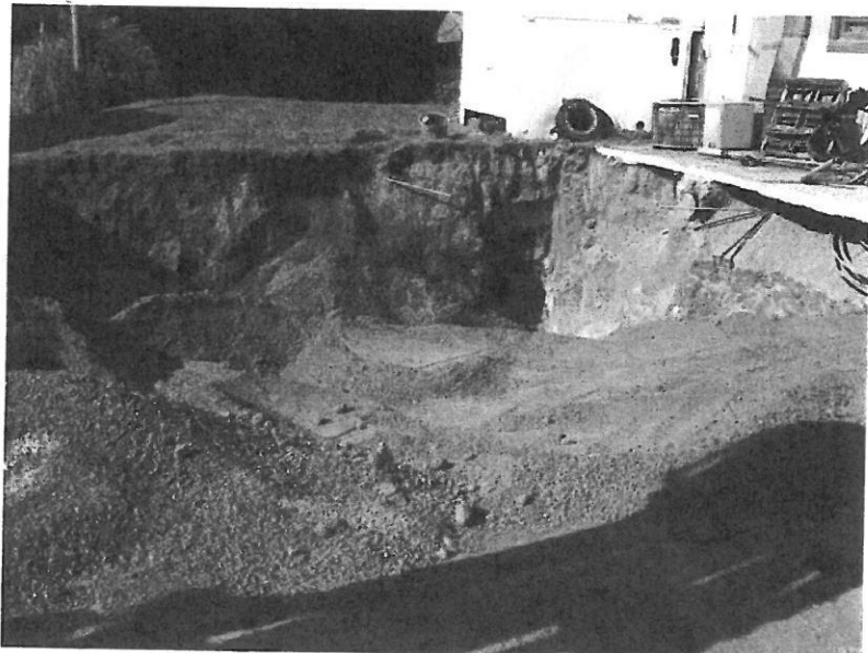
View showing backfilling of gasoline tank pit with pea gravel overburden.
