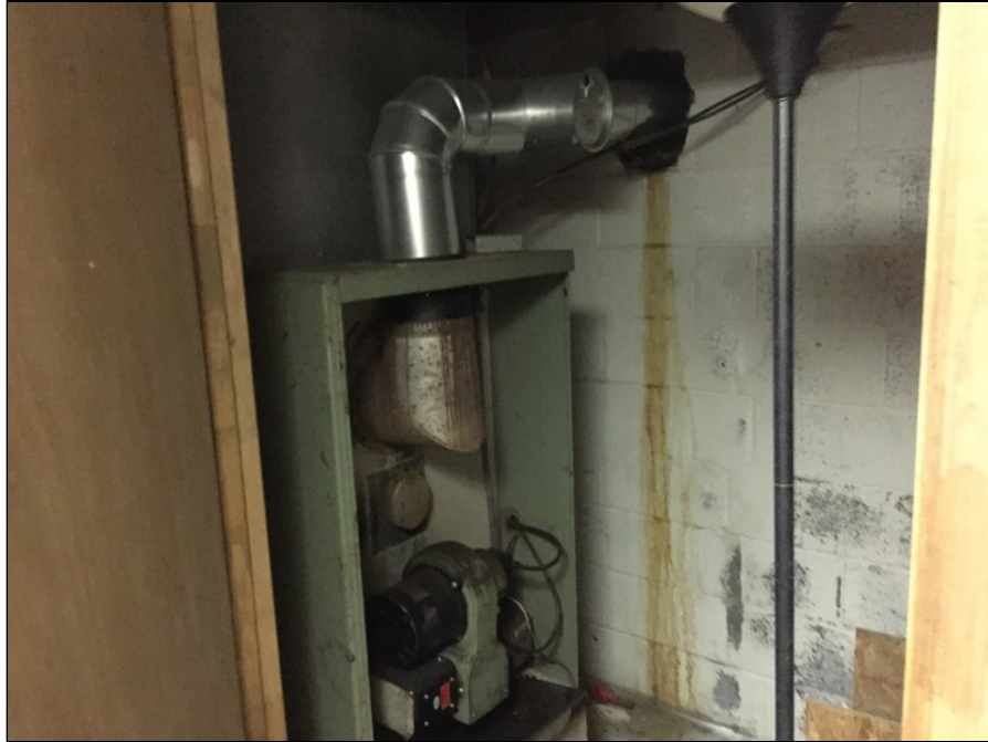
13 - Furnace in the convenience store that appears to be connect to the UST.
