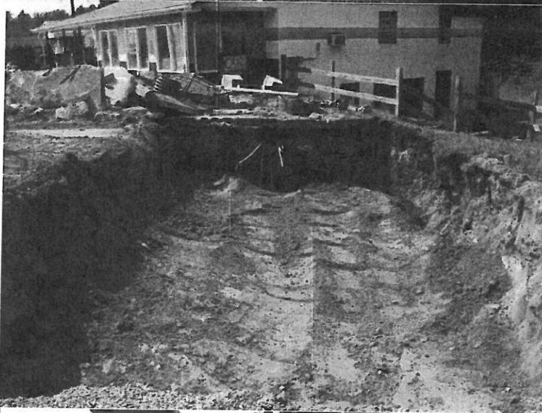
View showing diesel/kerosene tank pit bottom following backfill with overburden soil and pea gravel.
