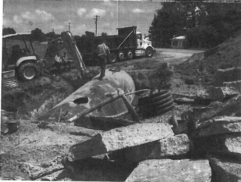
View showing diesel/kerosene tank following triple rinsing and interior cleaning.
