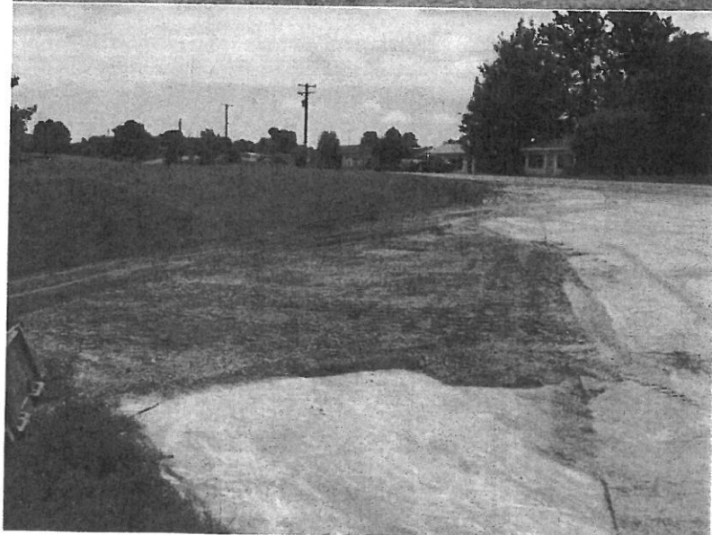
View showing top layer of ABC stone over diesel/kerosene tank pit.
