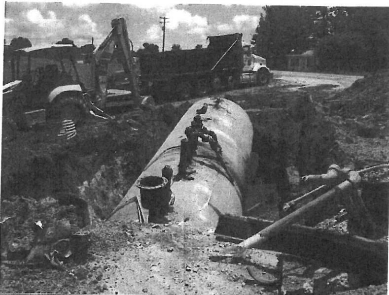
View showing diesel/kerosene tank after being broken free from pit bottom.
