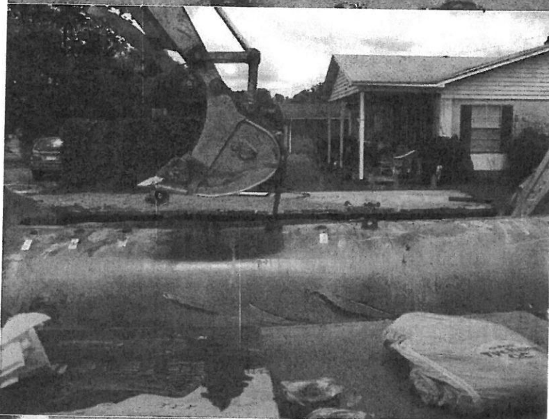
View showing first gasoline tank being broken free from pit bottom.
