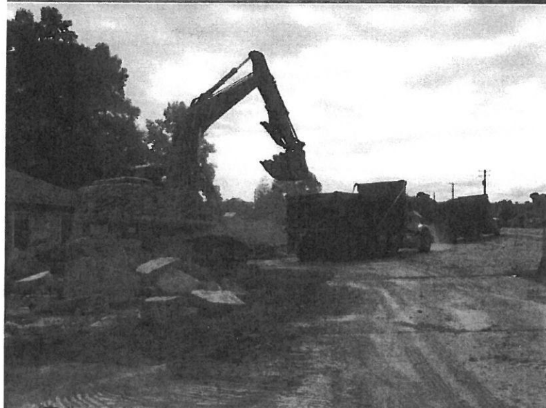
View showing concrete debris being loaded for transport and disposal off site.
