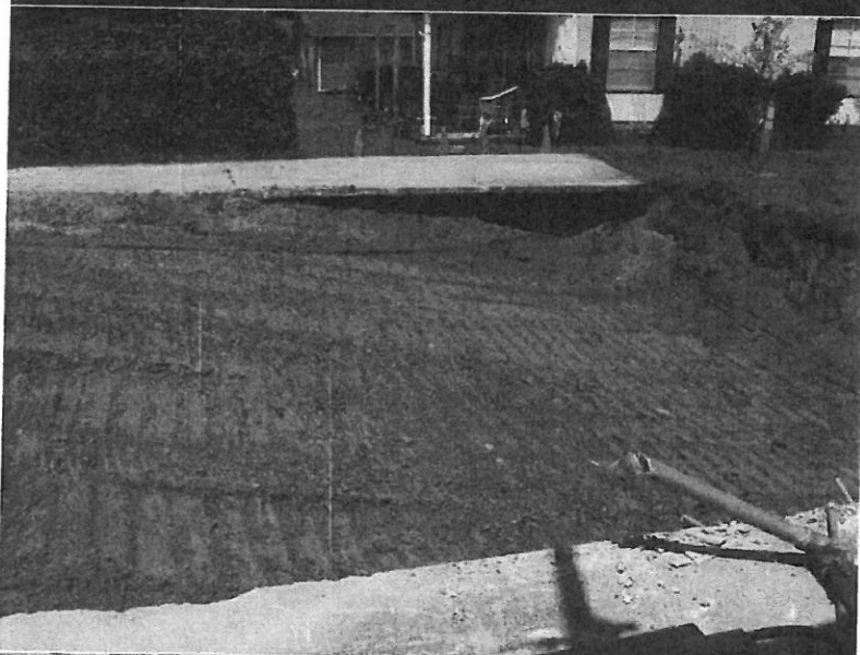
View showing gasoline tank pit backfill.
