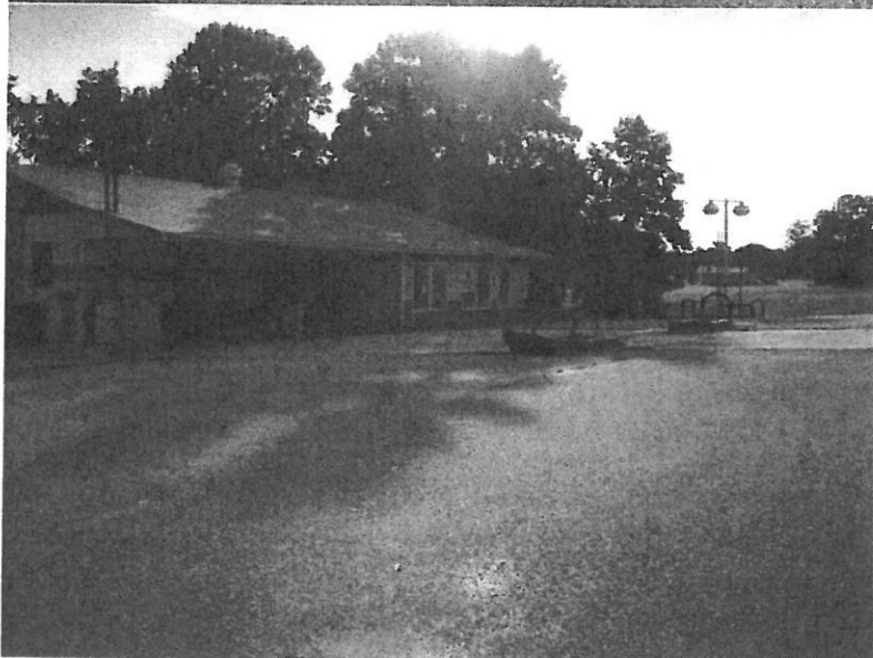
View across property from west side looking northeast prior to site UST removal work.
