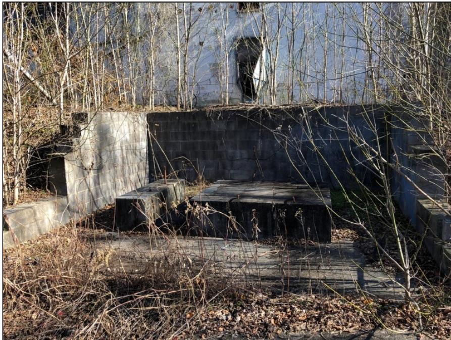
20 - View of what appears to be a former AST tank cradle.
