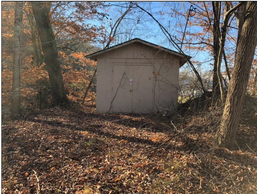
22 - Sprinkler pump house.
