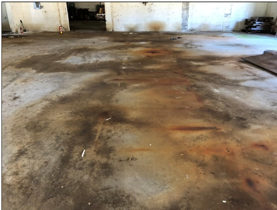
12 - Stained floor within the subject building.
