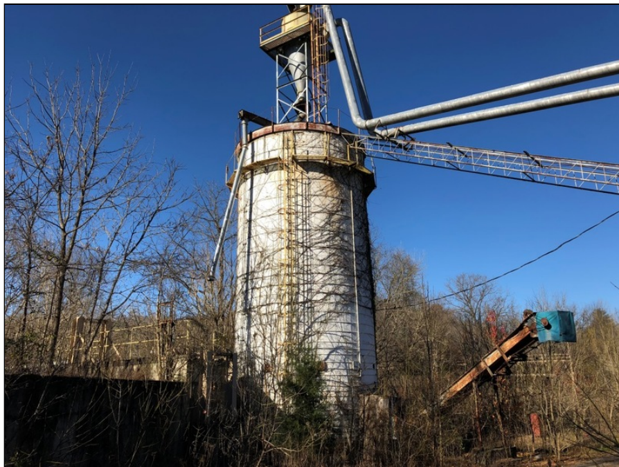
8 - Large silo on the western portion of the subject property.
