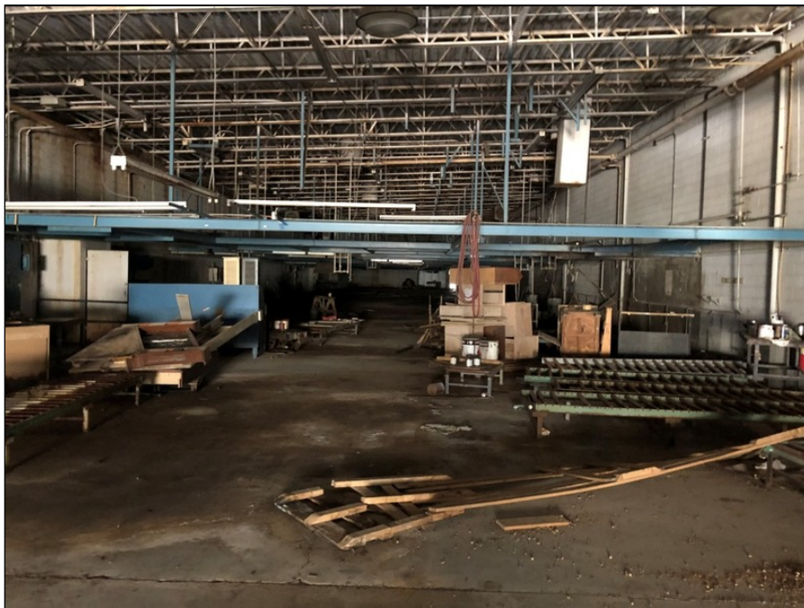
14 - Apparent production/manufacturing area within the subject building.
