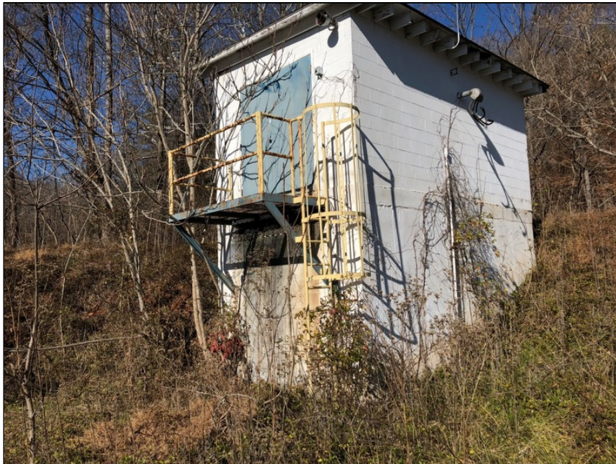
16 - Pump house on the northwestern portion of the property.
