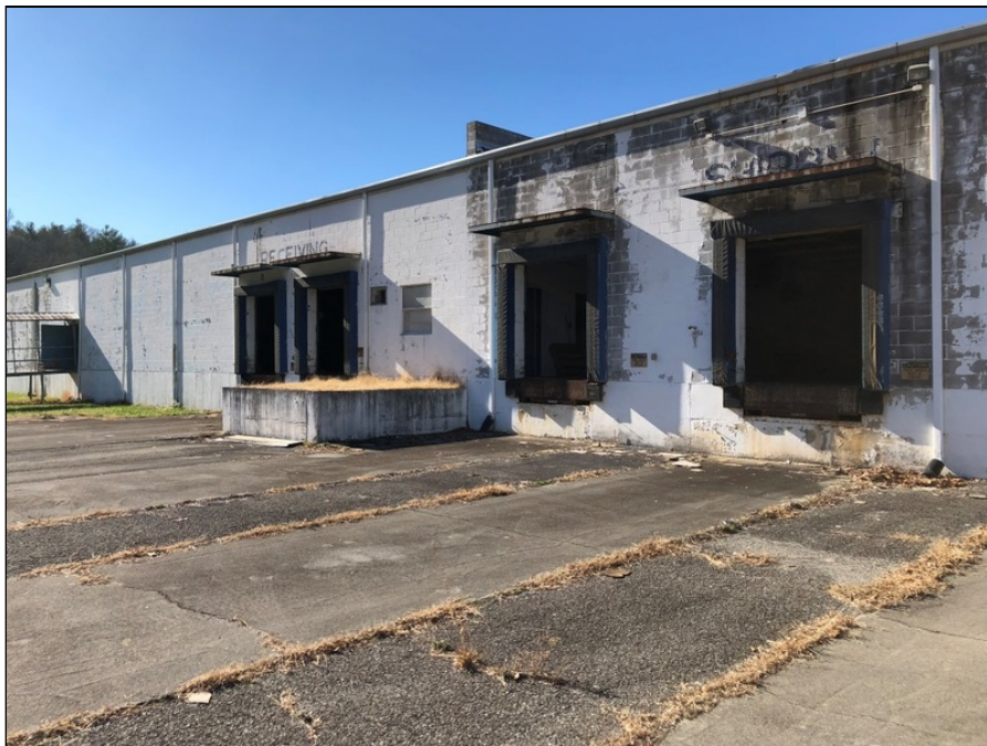
4 - Loading docks near the northeastern portion of the subject building.
