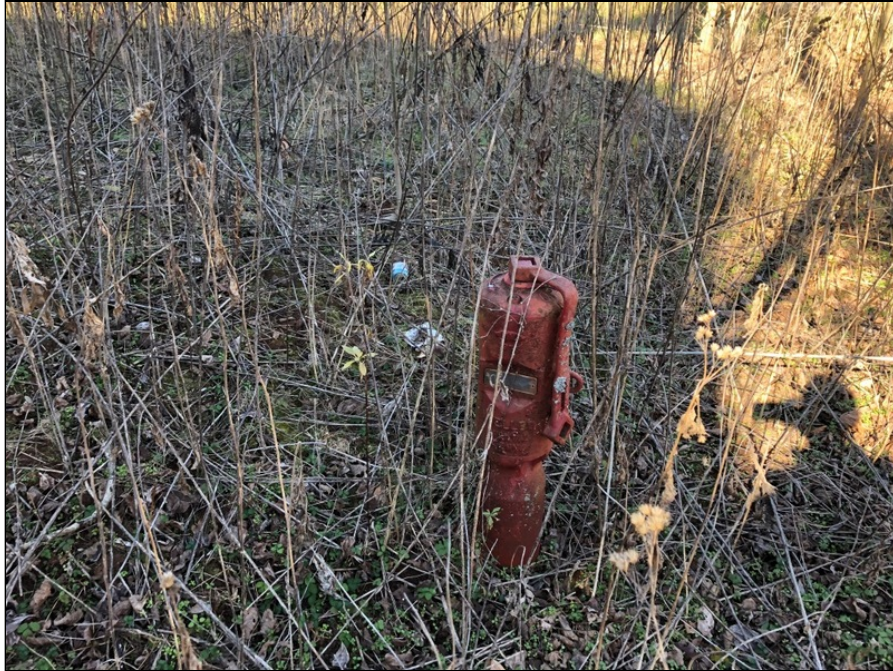
9 - Hydrant casings along the western portion of the property.
