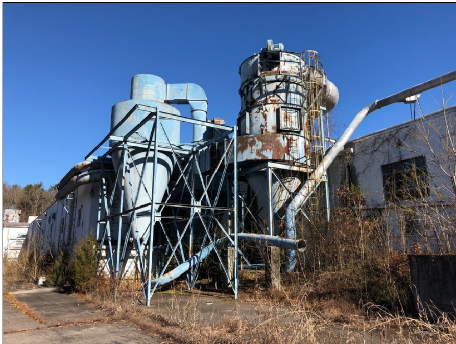
10 - Large hoppers on the western side of the subject building.
