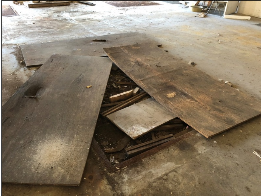
21 - Former inground equipment, likely a scale.
