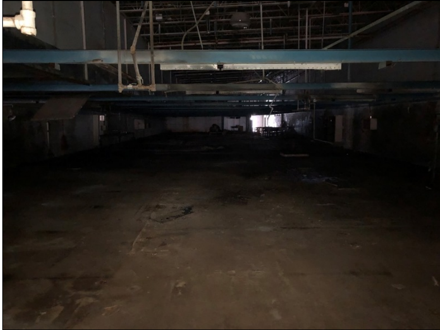
13 - Apparent production/manufacturing area within the subject building.
