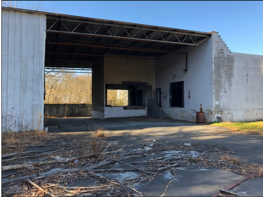
1 - Southern portion of the subject building ('drive-through loading area')
