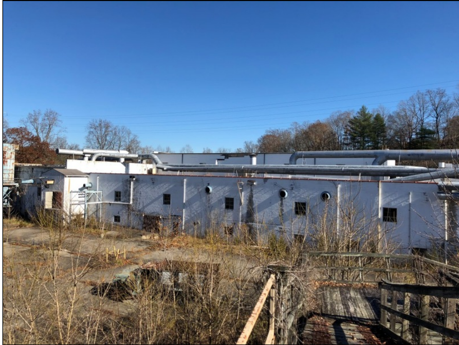
17 - The back of the subject building.
