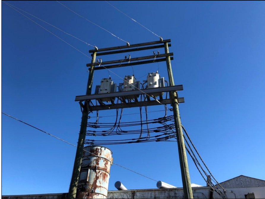
11 - Pole mounted transformers on the western portion of the subject building.
