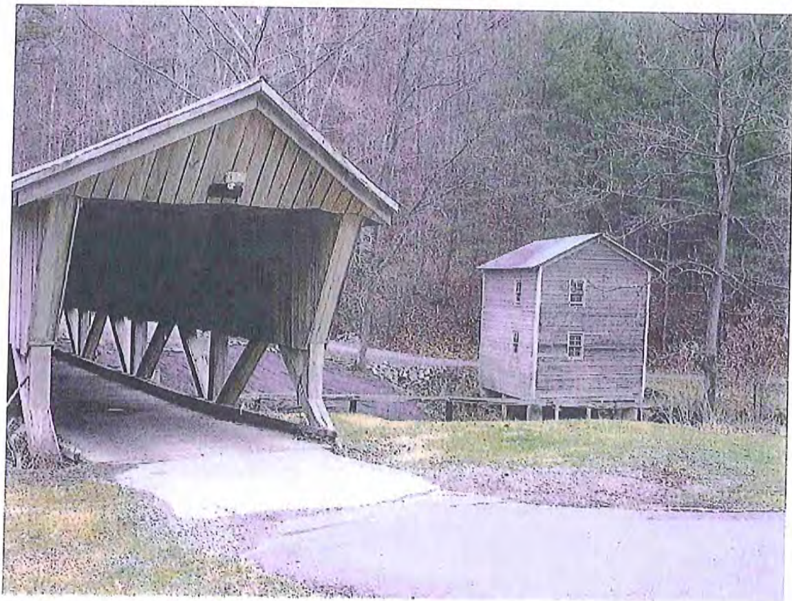
EXISTING COVERED BRIDGE AND MILL HOUSE
